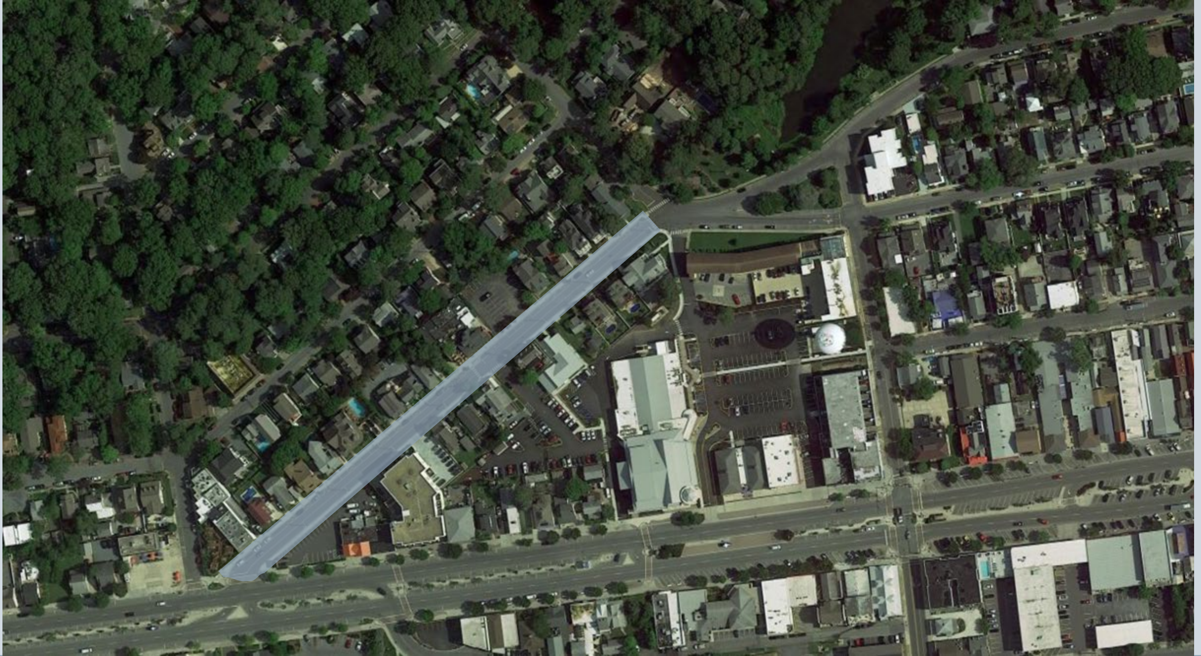
Lake Avenue Streetscape - Phase II
