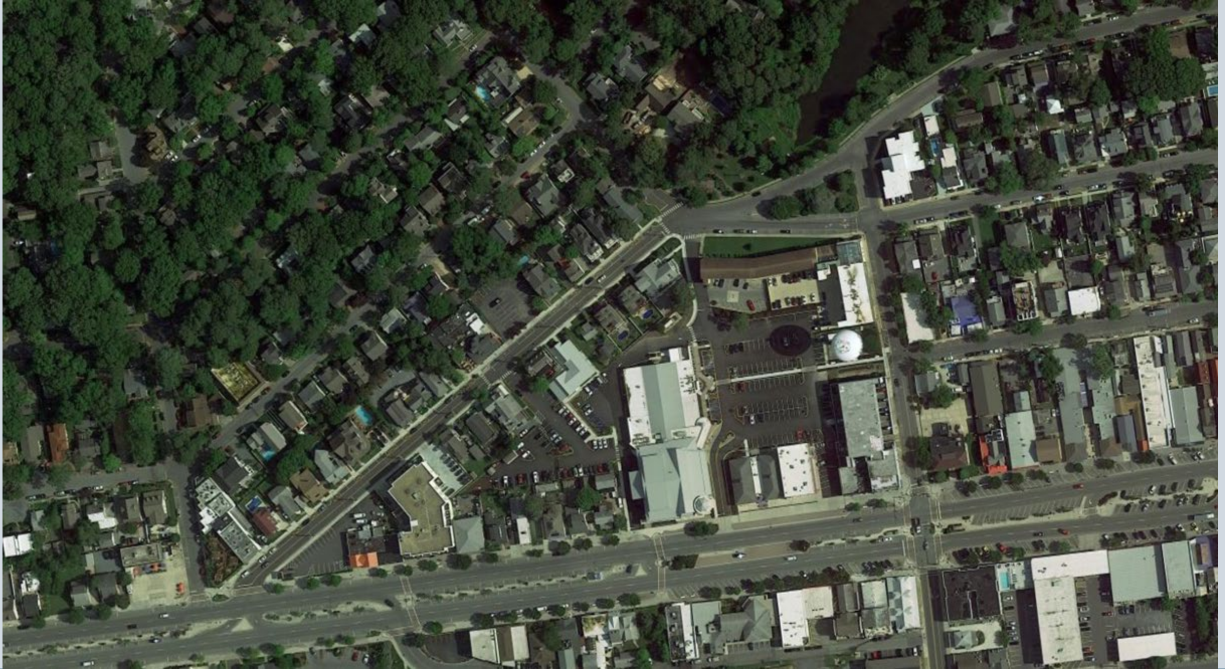
Lake Avenue Streetscape - Phase II
