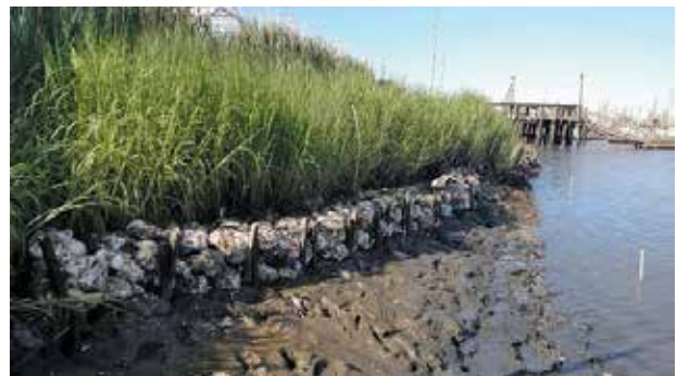
Recycled oyster shells are used to stabilize a shoreline.
