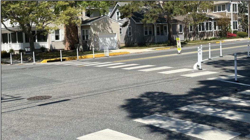
Bump outs at King Charles Avenue and New Castle Street.
