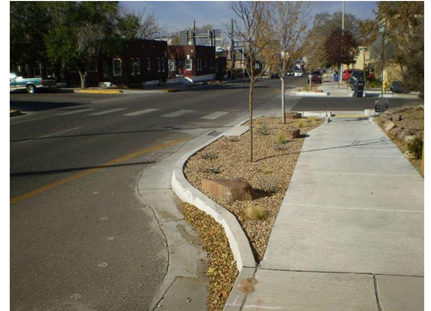
Permanent Bump Outs and Crosswalk Source: FHWA
