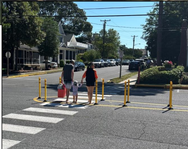
Refuge Island at King Charles Avenue and Stockley Street
