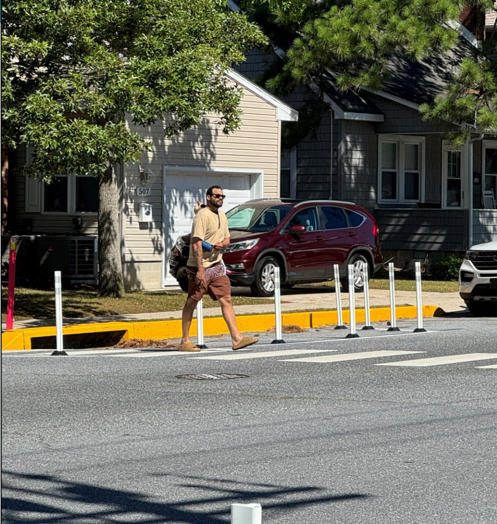
Bump outs at King Charles Avenue and New Castle Street.
