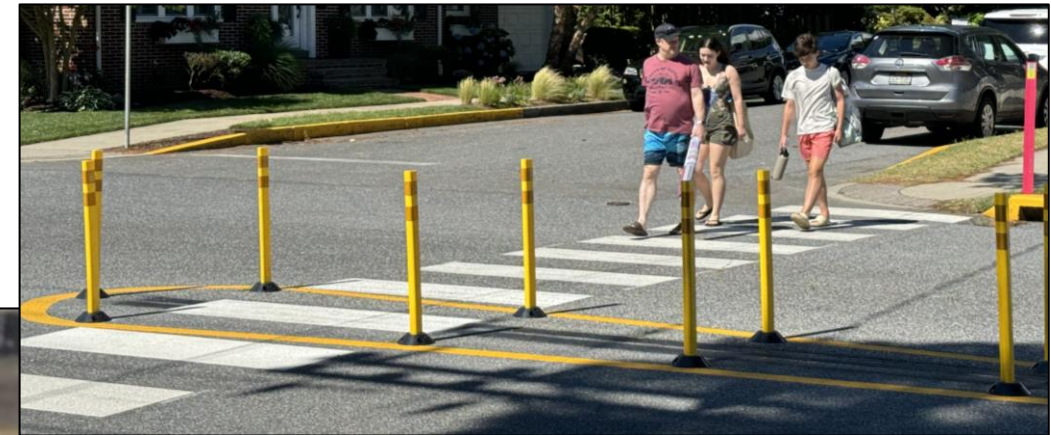
Flex Post Median Island at King Charles Avenue and Stockley Street
