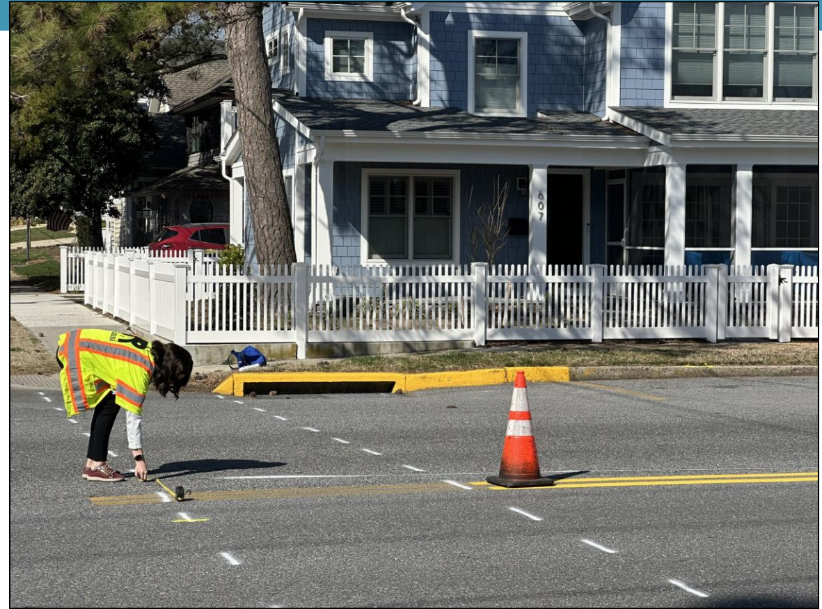
King Charles Avenue 3/14/24 Field Mark Up
