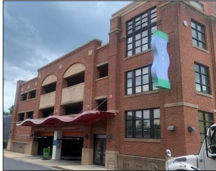
Knighton Garage, Annapolis, MD Source: visitannapolis.org
